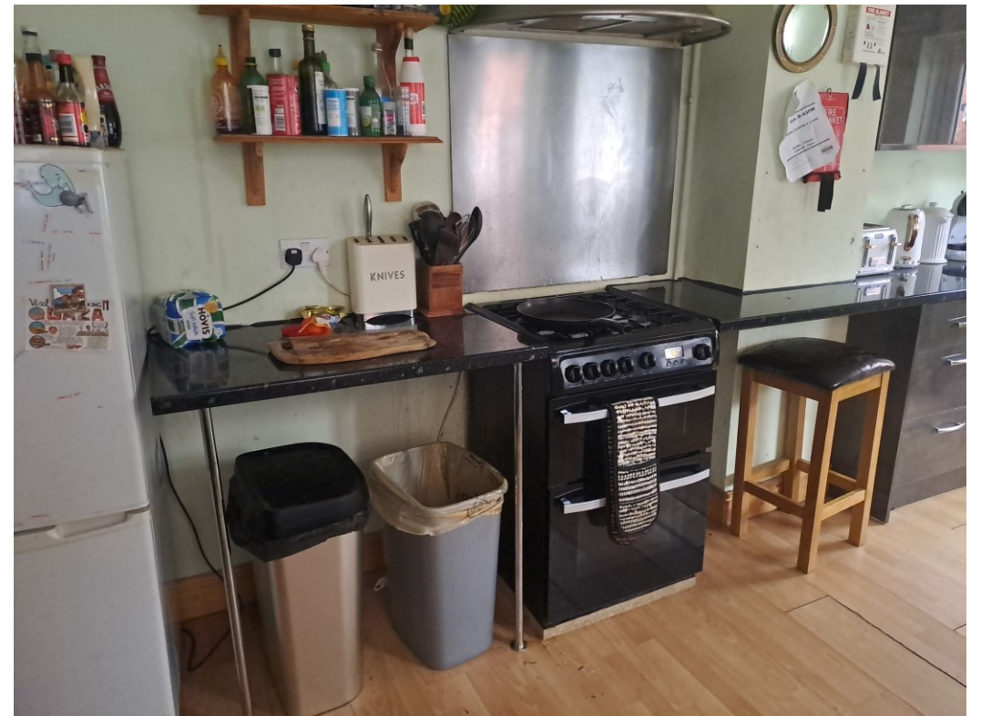
New worktop installed on both sides of the cooker
